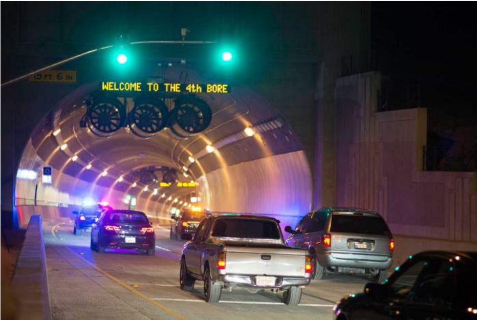
Caldecott Tunnel 4 th Bore
