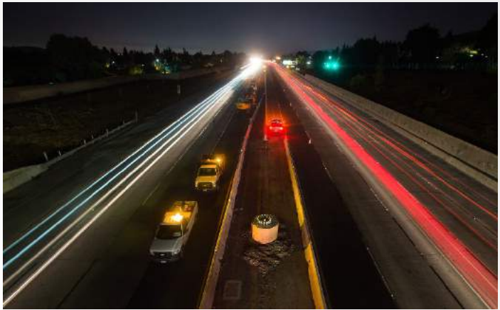
Express Lane Construction
